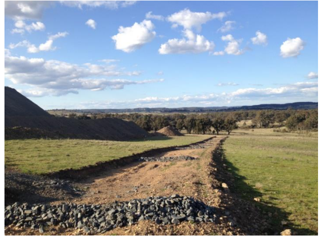
Plate 1 - Drainage Channels Around Existing Emplacement Area
