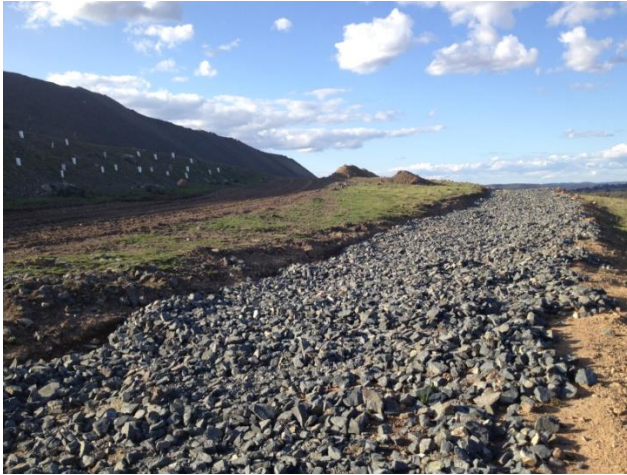
Plate 1 - Drainage Channels Around Existing Emplacement Area
