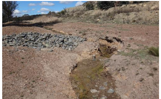
Photo 18- Dirty water channel extension below advancing emplacement
