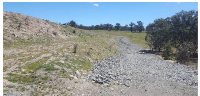
Photo 13- Protected Drainage Channel
