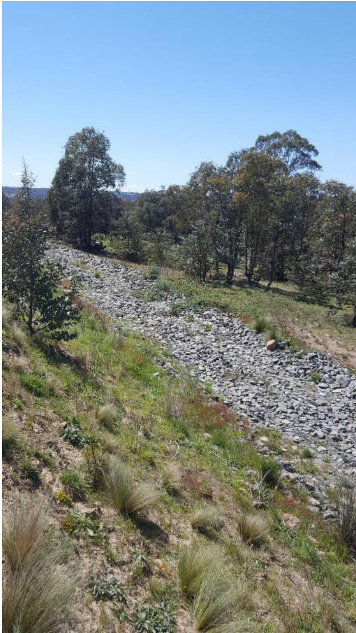
Photo 16 - Protection Channel in Older Rehabilitation Area
