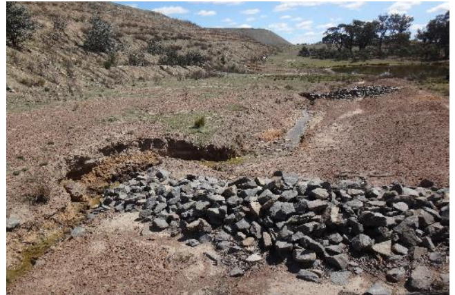
Photo 17- Dirty Water Channel with Check Dam Structures
