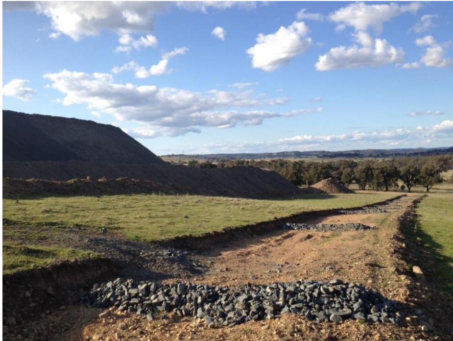
Plate 6 Rehabilitation of Bund Wall / Overburden Emplacement Area with Drain in Foreground
