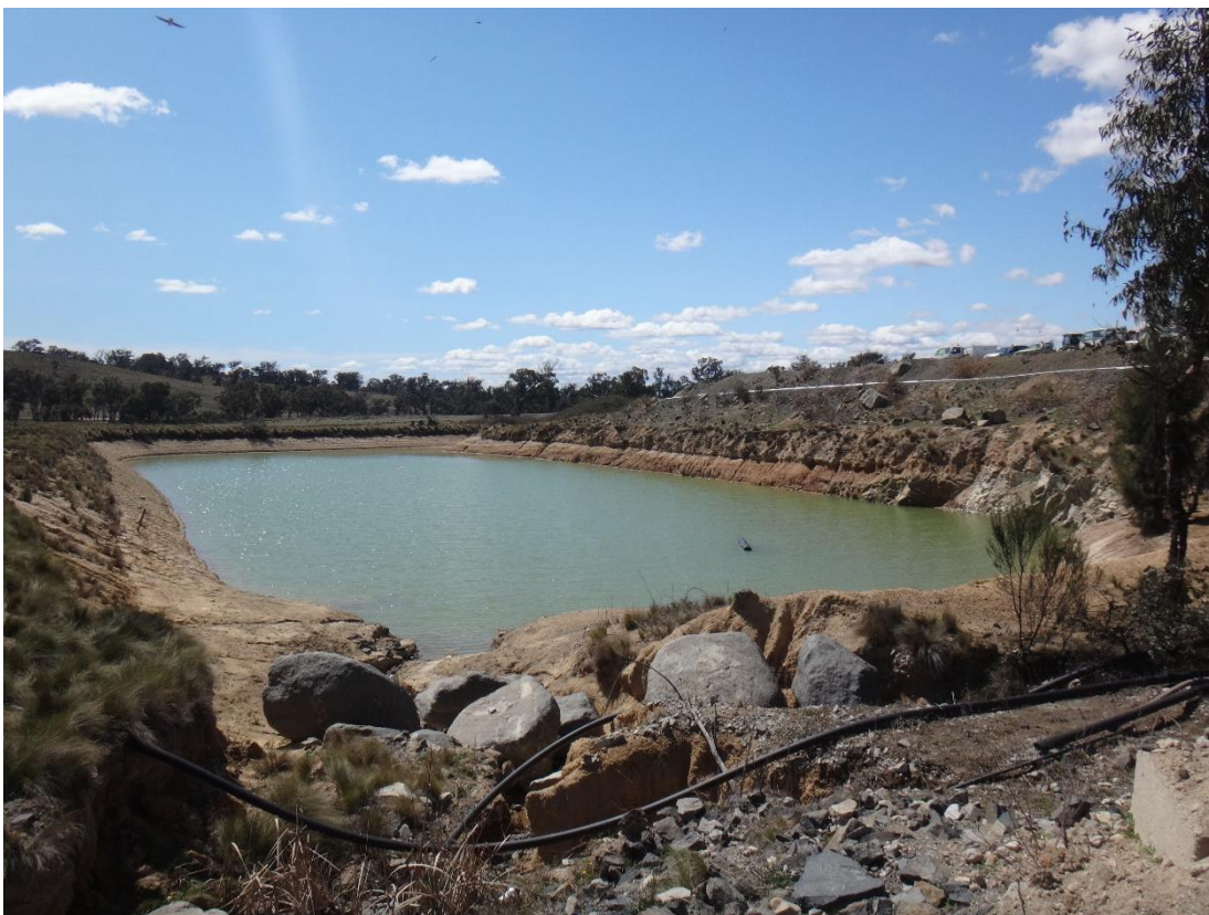
Plate 8 Process Water Dam
